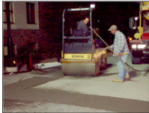
Figure 5 – Rolling Porous Concrete
