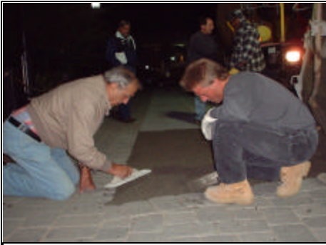
Figure 4 – Hand Trowling PC
