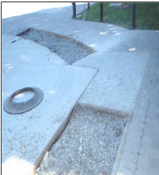
Figure 3 –Sections of removed PC
