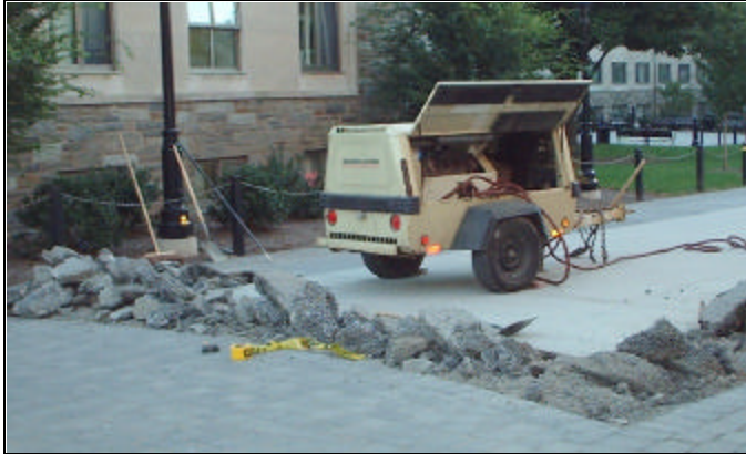
Figure 2 –Demolished Concrete on Upper Bed
