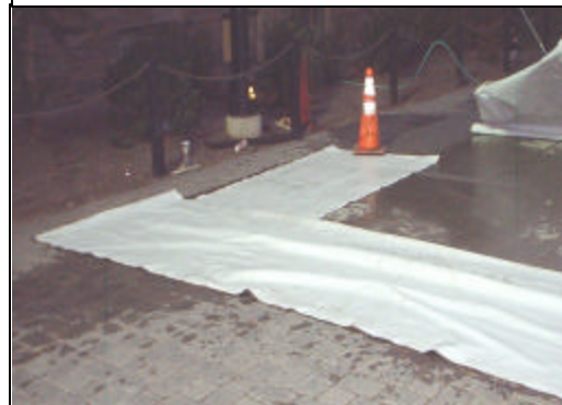
Figure 6 – Wet Burlap Covering
