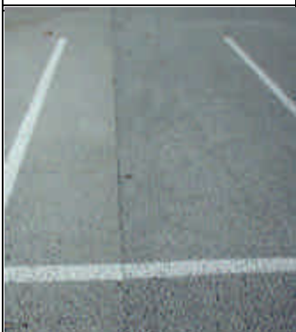
Figure 7 - UNC Parking Lot
