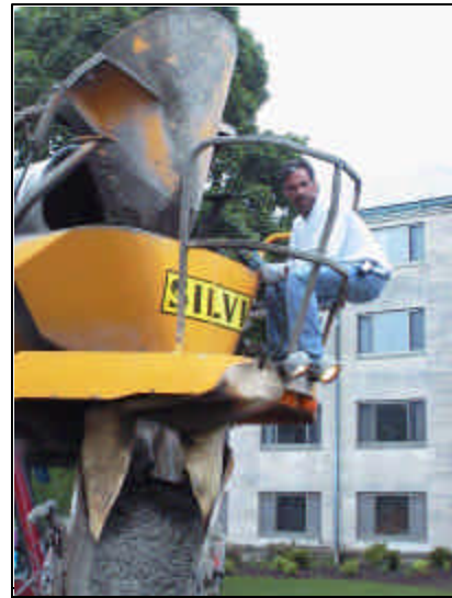
Figure 10 - Concrete Truck and Foreman
