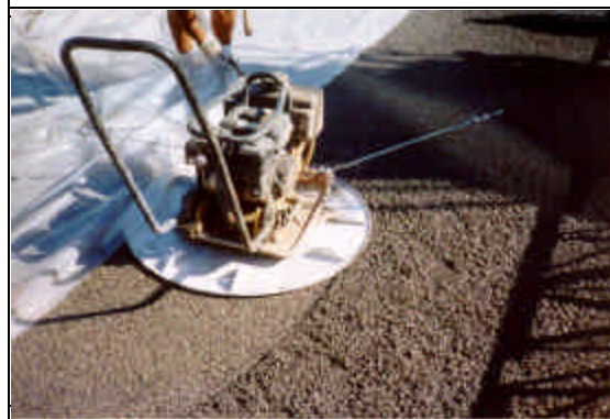
Figure 3 - Vibratory Tamping
